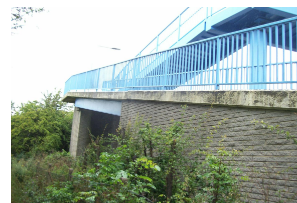
Photograph 8 South elevation of the ramp
