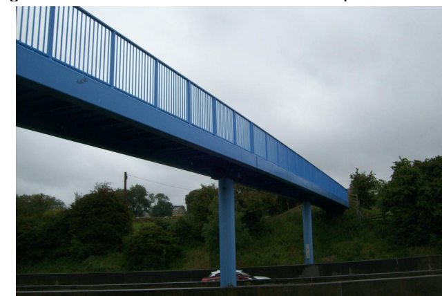
Photograph 9 South elevation of the footbridge
