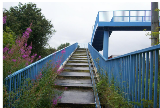
Photograph 7 View of the ramp
