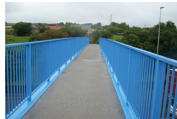
Photograph 5 View of surfacing on bridge deck
